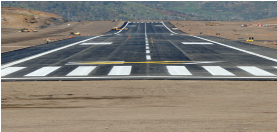
Telluride airport's newly renovated and much-improved runway.
